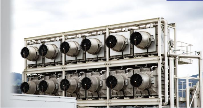
Capricorn was Climeworks' first direct air capture plant on an industrial scale.
